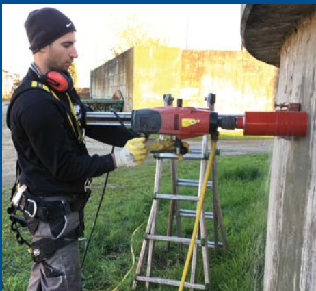
the tripod-guided core drilling machine using a wet drilling process
