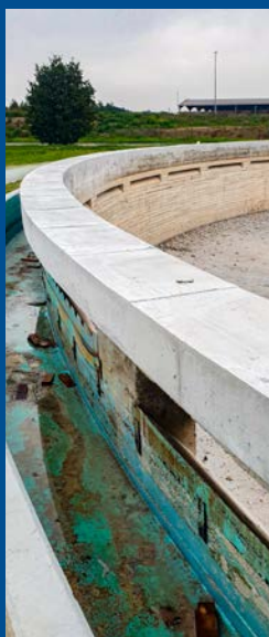
Reggio Emilia, Italy / extensive concrete refurbishment and scraper tank track
