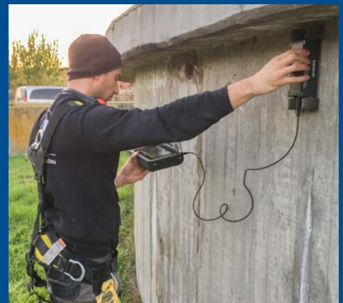
scan of reinforcement to determine the reinforcement positions and concrete covering
