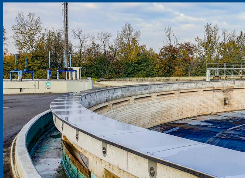
Reggio Emilia, Italy / extensive concrete refurbishment and scraper tank track
