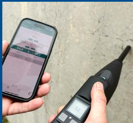
testing the compressive strength
