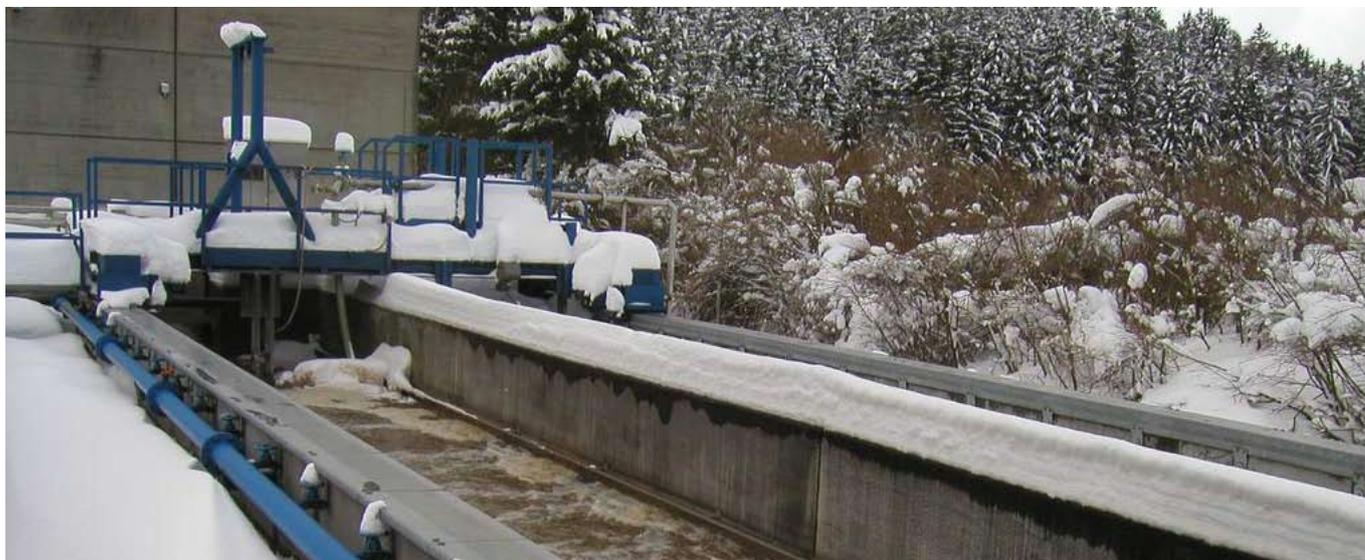
Clearly, a heated scraper runway simplifies the winter operation considerably. What is new about this is that the operating costs of such a heating system are next to nothing because one can dispense with external energy sources. Both pictures show this type of installation; last winter we undertook several extensive tests and the product proved itself superbly. Innovative technology from Krumme GmbH! We will gladly inform you about our products!
